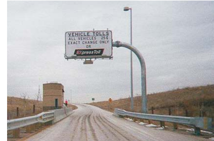
Tollway Highway with access only at grade-separated interchanges and no at-grade intersections. User tolls required.
