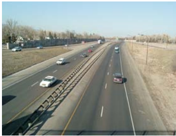
Freeway Highway with access only at grade-separated interchanges, no at-grade intersections.
