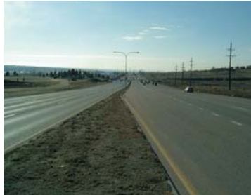
Enhanced Expressway A limited access arterial highway which contains both at-grade intersections and grade-separated interchanges. "Enhanced" refers to a higher proportion of interchanges than intersections, which results in increased capacity. The highest-volume intersection locations are converted to grade-separated interchanges.
