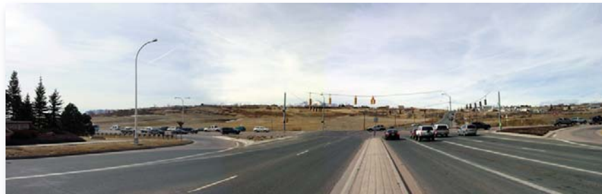
Existing: Barnes looking west
